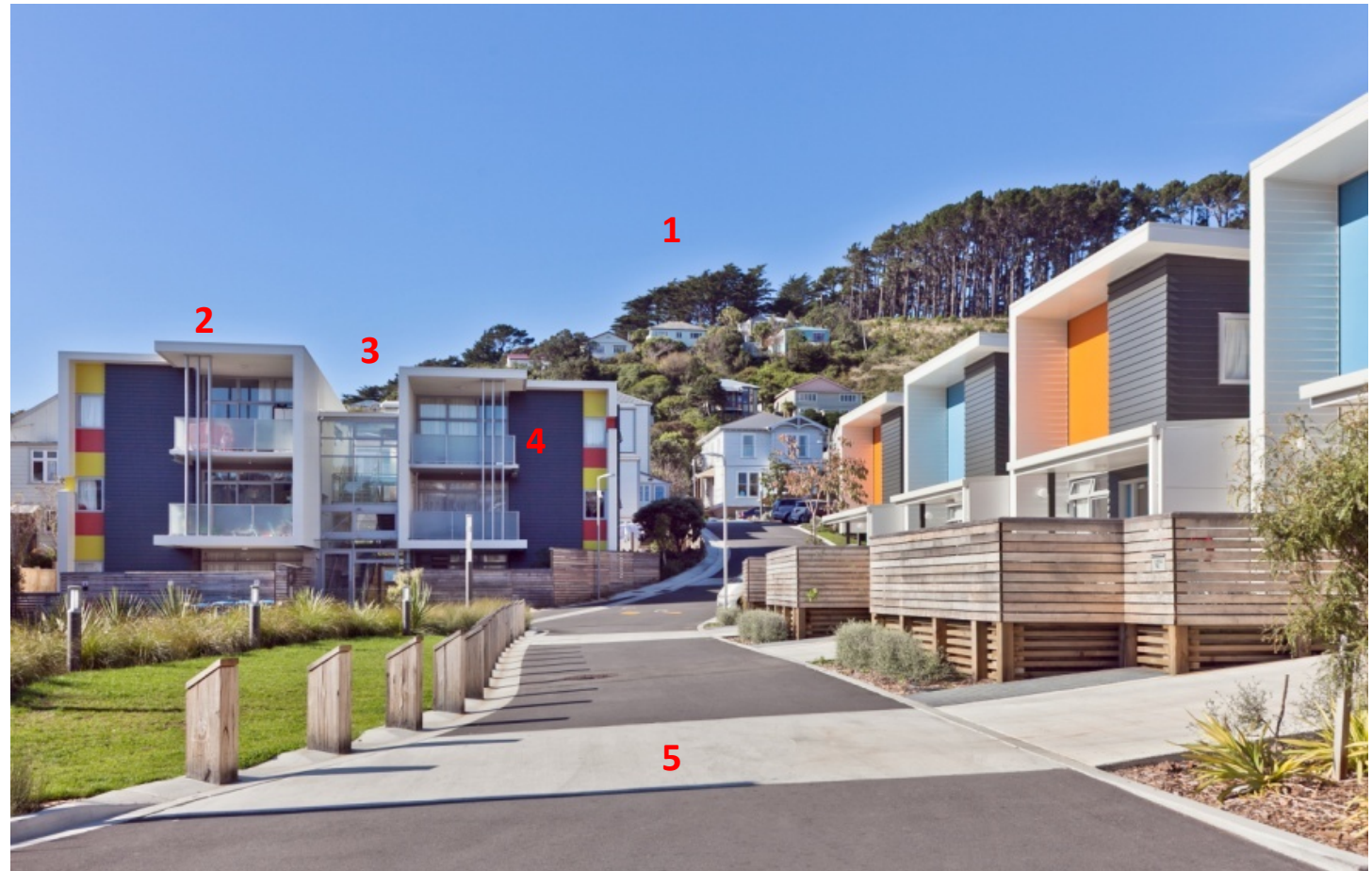
Looking towards the main entrance to the site which is from Owen Street.
