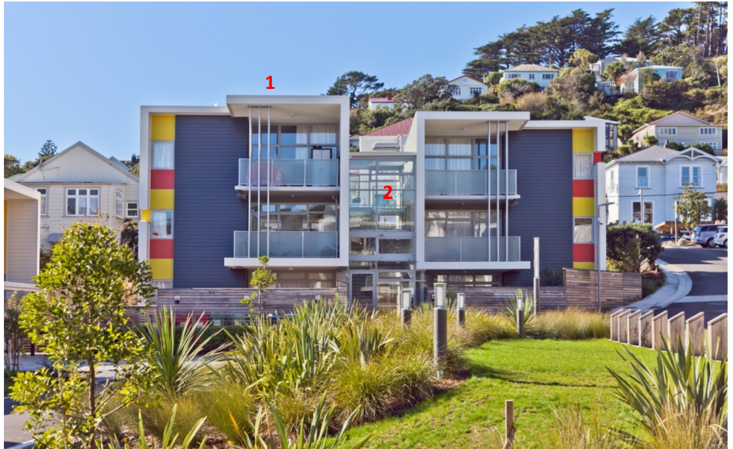
View of a typical apartment block – These apartments presents an attractive interface to Owen Street.
